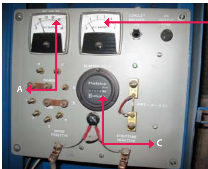
Photo 7: A common rectifier for an impressed current cathodic protection system. The photo shows the volt meter (A) and ampere meter (B). Neither meter should read zero if the rectifier is functioning properly. Some rectifiers also have an hour meter (C).
