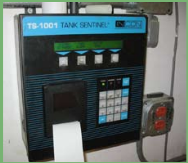
Photo 1: Examples of Automatic Tank Gauges (ATGs).
