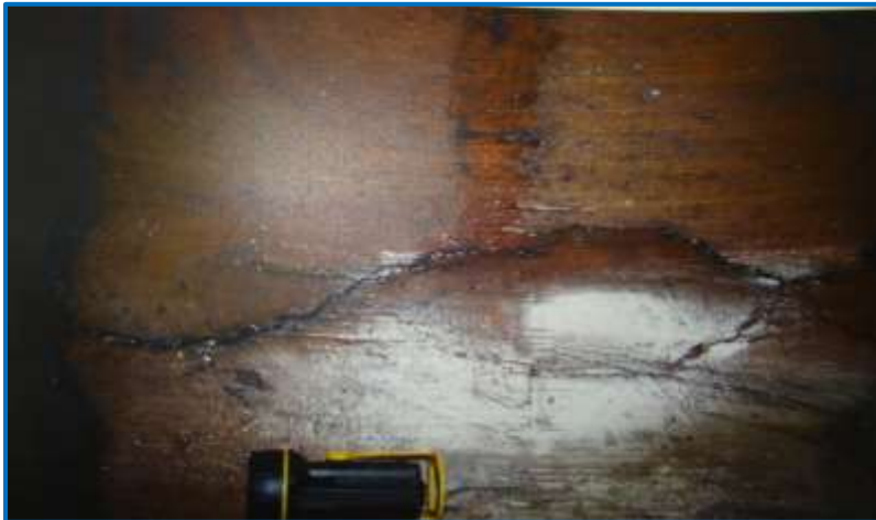
92 Octane UST interior – water entering tank through crack
