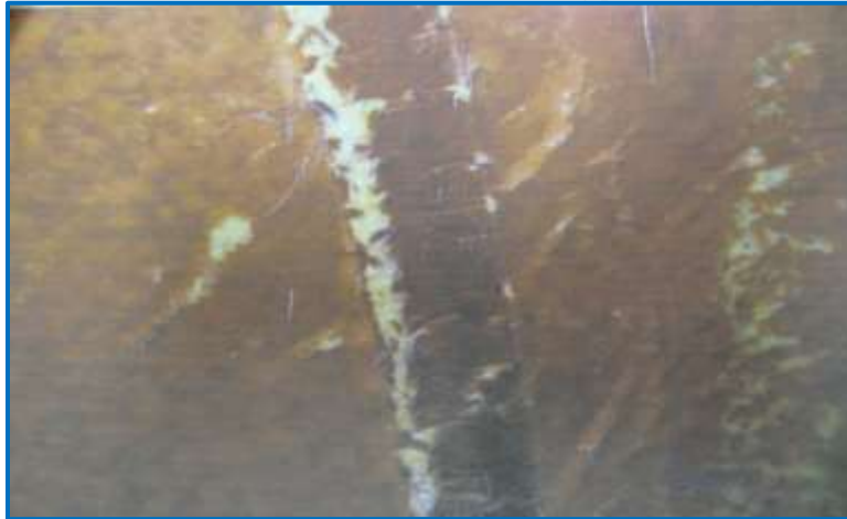
92 Octane UST – breakdown observed during pre-blast inspection
