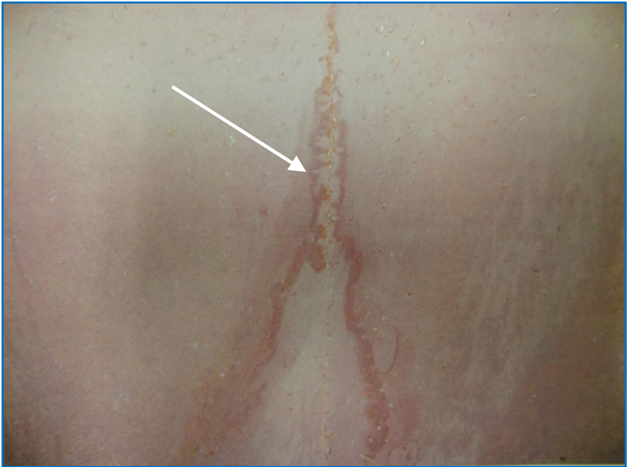
UST 89 Octane internal view: crack
