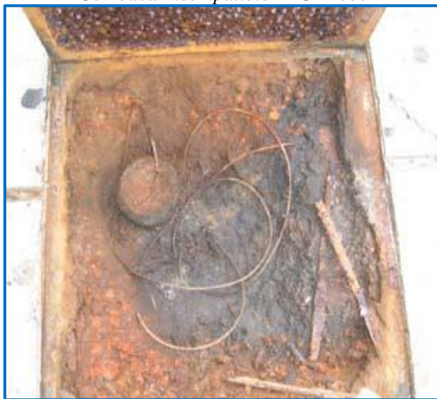
Corroded Incompatible ATG Probe
