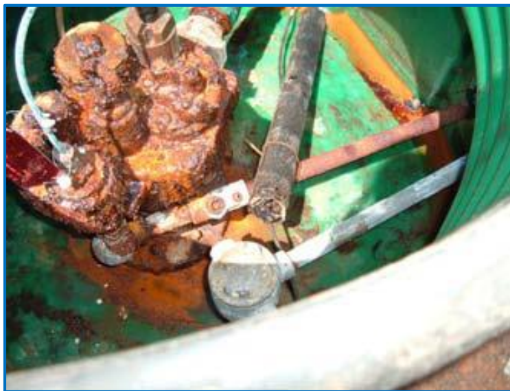
Corroded STP
