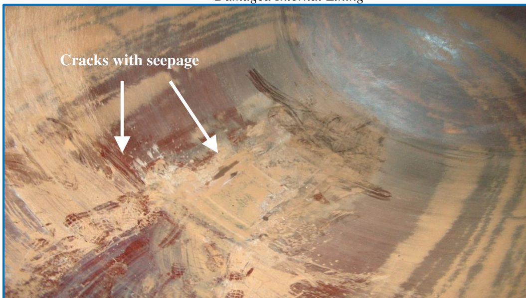
Supporting Pictures: Damaged Internal Lining
