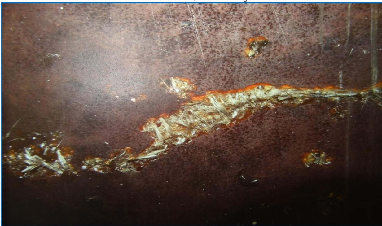
UST 92 Octane interior view: horizontal cracking in tank shell
