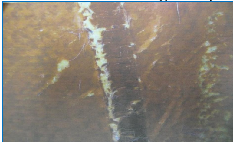
92 Octane UST – breakdown observed during pre-blast inspection
