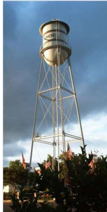
This steel tank in Raymond, Mississippi, has been in continuous use since 1905.
