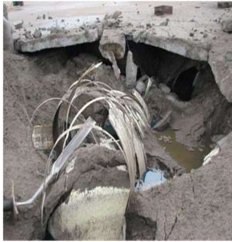
Steel is naturally grounded. A steel tank won't explode like this FRP tank did when lightning struck nearby.
