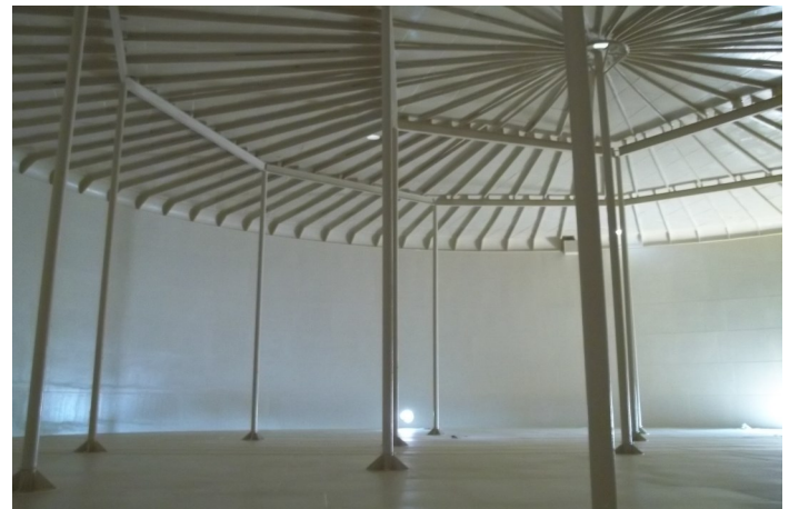
Inside Coating System 4: Zero VOC Epoxy (ICS No. 4)
