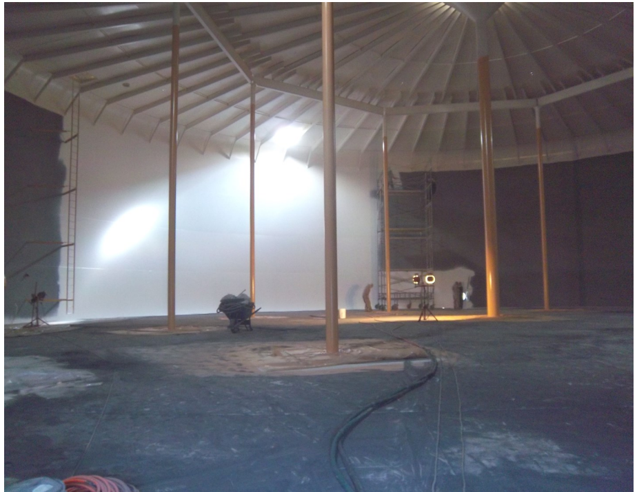
Inside Coating System 3 : Zero VOC Polyurethane (ICS No. 3)
