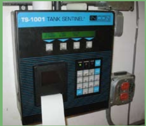
Photo 1: Examples of Automatic Tank Gauges (ATGs).
