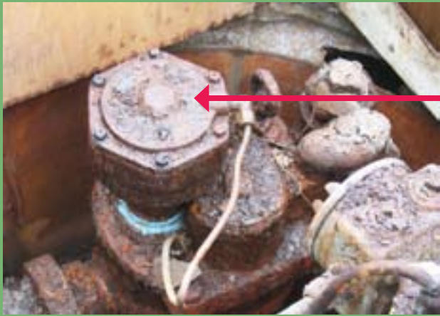
Photo 4: Different examples of mechanical line leak detectors (MLLDs).
