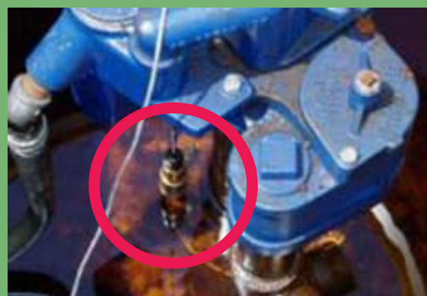
Photo 6: Examples of sump sensors.
