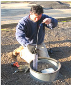
David Ellis of Lighthouse Electric Technologies Installing Liquid Sensors
