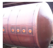
Permatank in North Carolina
