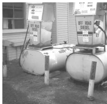
What's wrong with this picture?
