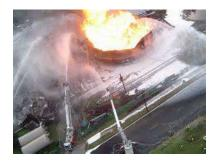
Small fires radiate less heat and, for fuels with high percentages of alcohol like E85, even less thermal energy is generated. That assumption is accurate for small fires, but not fires in large ethanol storage tanks.
