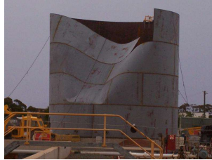
The picture above shows the effect of wind on a large tank that was damaged overnight during the construction phase.
