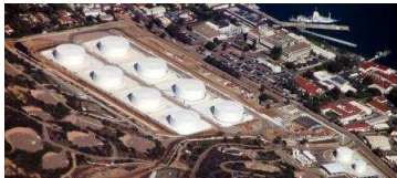
API Flat Bottom Oil Storage by CBI Services, Everett WA.
