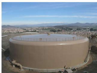
Flat bottom reservoir storage tank. Photo courtesy Paso Robles Tank, Paso Robles CA
