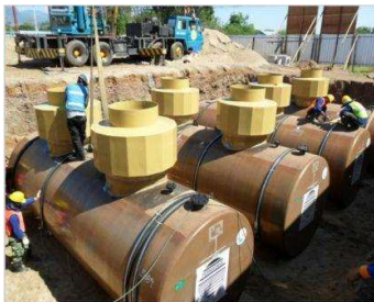
Permatank installation in Asia. Photo courtesy Padungsilpa Engineering, Thailand
