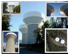
Two 3 Million Gallon W ater Storage Tanks by Caldwell Tanks, Louisville KY
