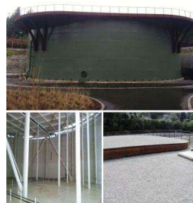
2.6 Million Gallon Reservoir Tank by Paso Robles Tank, Paso Robles CA.
