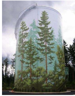
3 Million Gallon Standpipe by CBI Services, Everett WA
