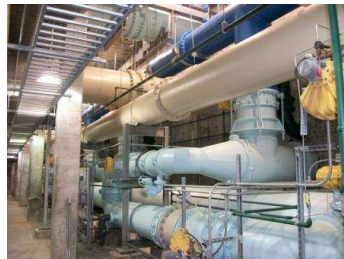
Steel Pipe Water Filter Gallery by MidAmerica Piping & Supply, Scammon KS
