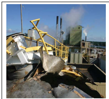
Source: CSB website - Views of the storage tank involved in the 2008 explosion at Packaging Corporation of America.
