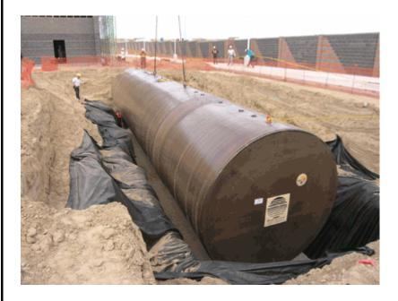
The West Side Transit Facility called for Permatank last year to meet a unique storage challenge. Serving buses in the local mass-transit district, the facility needed underground storage capacity for both fleet fueling and a backup-generator system.
