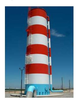
Among Standpipe entries, a 180,000-gallon (681,173 liters) tank for the Semitropic Water Storage District in Wasco, Calif. received the nod. Built by CB&I Constructors Inc. of San Luis Obispo, Calif., the 80-foot-high (24.38 meters) standpipe featured an aviation paint motif. Also included in the design was a ladder and cage system to provide safety when climbing, and an external overflow pipe to grade.
