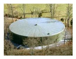
In the Reservoir category, a 5-million-gallon (18,921,000 liters) tank fabricated for Huntsville Utilities in Huntsville, Ala. received the top honor. Assembled by Fisher Tank of Cropwell, Ala., the project featured a solid slab foundation to span potential sinkholes and an all-welded 32-foot-high (9.75 meters) radial cone roof, including rafters, girders, plates and connections.
