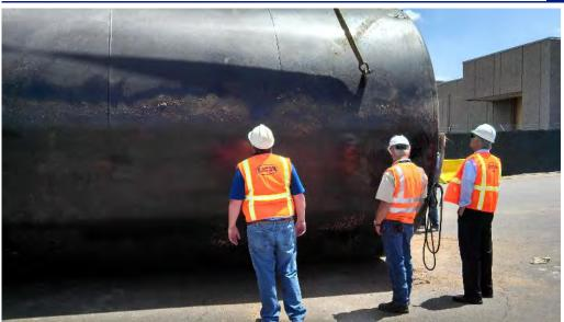
Eaton Metal Products, an STI/SPFA member, built six sti-P3 underground storage tanks in 1986. Recently, the tanks were removed by the owner and were found to be in excellent condition.
