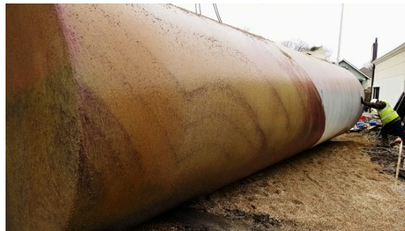
The tank was in excellent condition, with the fiberglass coating intact.
