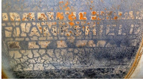
Flameshield label still visible after 24-36 hour site fire
