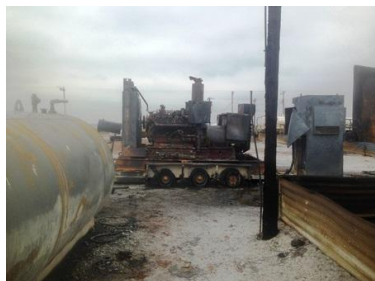
Fireguard tank (left) at fire site
