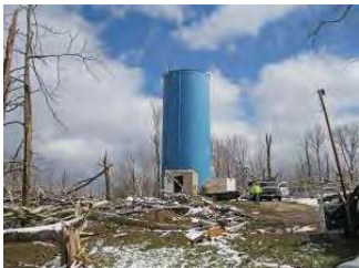
Photo: Bruce Cunningham, South Harrison (Indiana) Water Corp.
