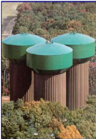
Left to right: single-pedestal spheroid tank (Wheaton, Ill.); three single-pedestal, fluted-column tanks (Bowie, Md.); composite elevated tank (El Paso, Texas); multi-column elevated tank (Beebe, Ark.)
