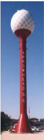
Left to right: single-pedestal spheroid tank (Wheaton, Ill.); three single-pedestal, fluted-column tanks (Bowie, Md.); composite elevated tank (El Paso, Texas); multi-column elevated tank (Beebe, Ark.)
