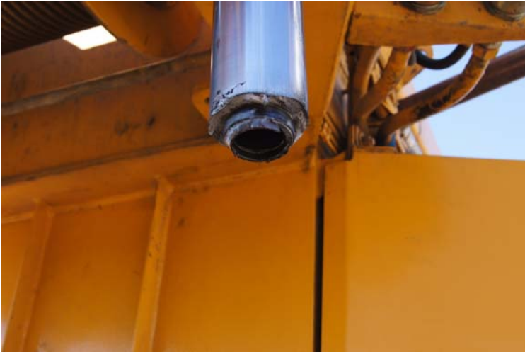
Close up view of hydraulic ram at north side of crane. End triangular locking piece has broken off
