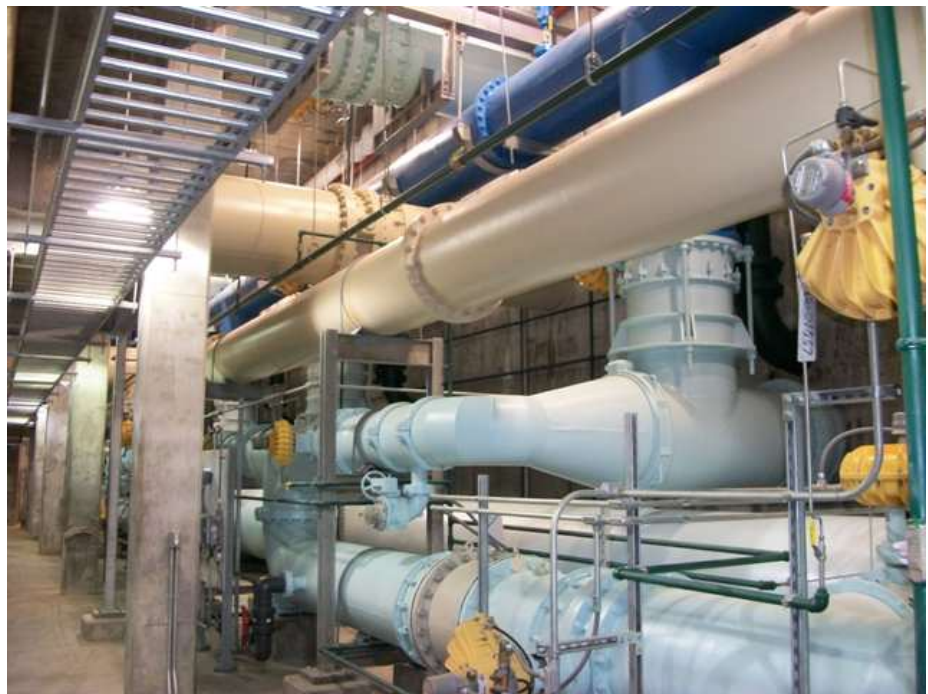
2012 Steel Pipe Fabrication of the Year Award Mid America Pipe Fabrication and Supply, LLC. Click here for description of Mid America's winning entry.
