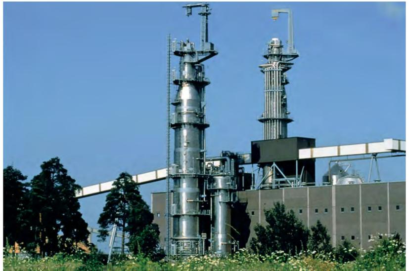
2205 continuous sulphate pulp digester and impregnation tower, Sodra Cell Mönsterås, Sweden (Source: Kvaerner Pulping)
