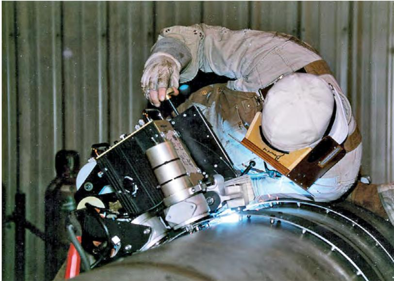
**Mechanized welding of large diameter duplex stainless steel pipeline on Alaska's north slope (Source: Arco Exploration and Production Technology)**
