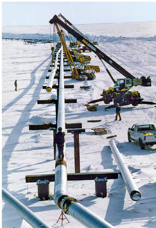
**Installation of insulated 24 inch 2205 pipe on vertical support members in Prudhoe Bay (Source: Arco Exploration and Production Technology)**
