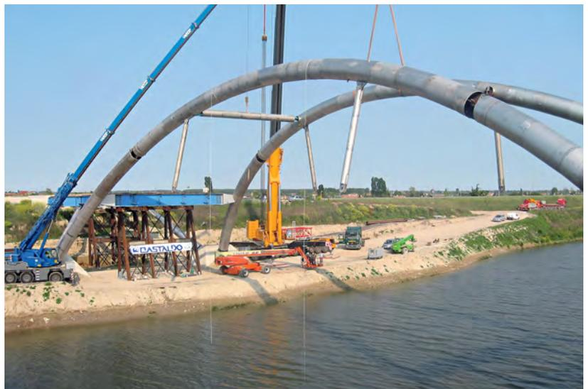
2304 duplex stainless steel bridge arches in construction near Padova, Italy (Source: ArcelorMittal)
