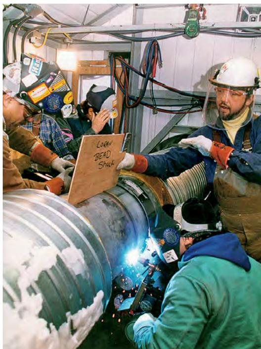
**Mechanized welding of large diameter duplex stainless steel cross-country pipeline (Source: Arco Exploration and Production Technology)**
