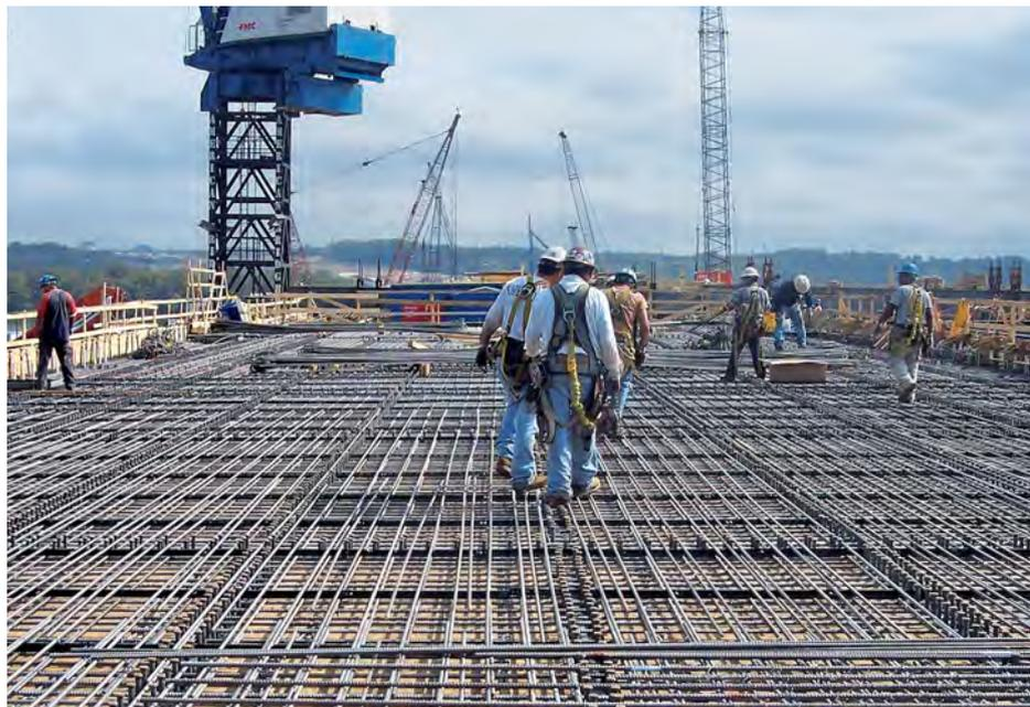
**Installation of duplex stainless steel rebar on a large bridge deck (Source: Hardesty & Hanover, LLP)**
