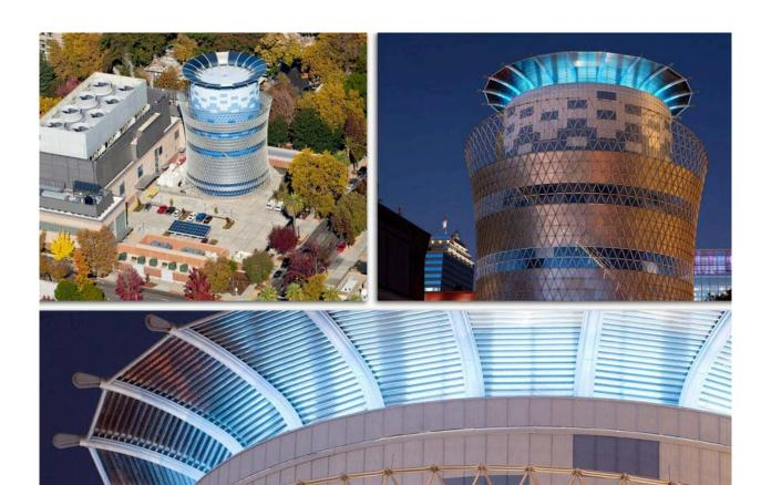
This is a one of a kind 4,000,000 Gallon welded steel Standpipe that operates as a 140' tall thermal energy storage (TES) tank built for the State of California's Central Utility Plant in Sacramento.
