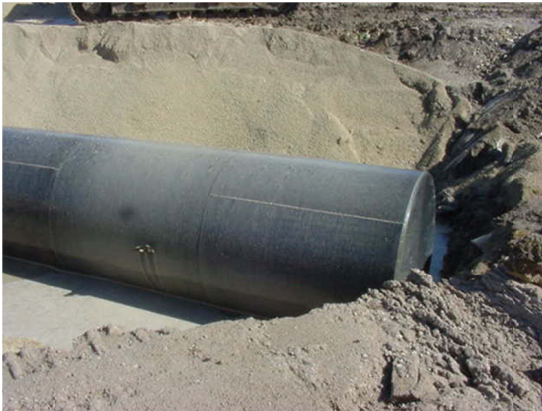
Picture 8 - Exhumed Tank After Test
