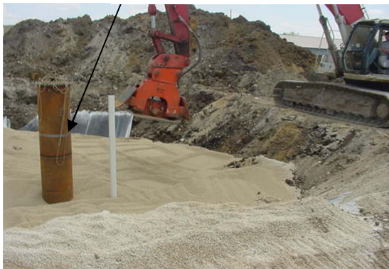
Pictures 3 & 4 - Vibratory Plate Utilized for Backfill Consolidation
