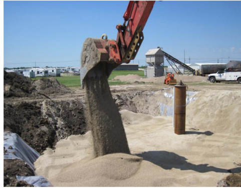
Picture 2 - Placing backfill over tank
