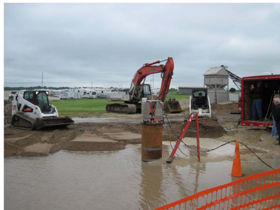
Picture 6 - Finished Backfill & Water at Ground Surface
