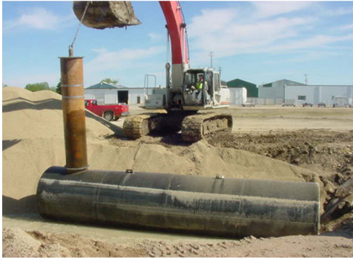
Picture 1 - Setting Tank on Bedding
