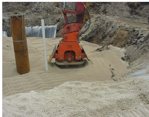
Pictures 3 & 4 - Vibratory Plate Utilized for Backfill Consolidation
