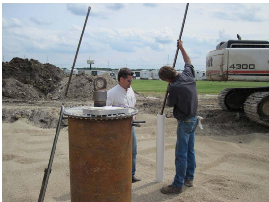
Picture 5 - Ground Water Level Verified
