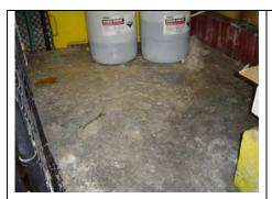
Chemical storage area floor is uneven as a result of chemical reactions, creating a slip and fall hazard.
