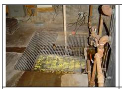
Exposed floor hole at sump pit in basement.
