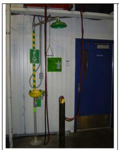
Battery charging station located directly above and adjacent to eye wash station and emergency shower. This is an electrical hazard near water sources and it appears that when the batteries are being charged, the eye wash station and emergency shower would be blocked and inaccessible. Additionally, the flexible cords appear to be passing through the doorway to the other side on a regular basis.
