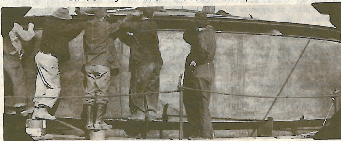
GATX Tank Erection Corporation installing petroleum Lifter Roof Tank
